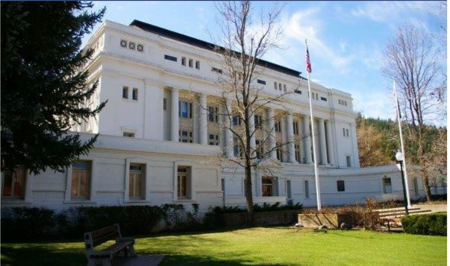
The Quincy Courthouse for the Superior Court of California, County of Plumas
